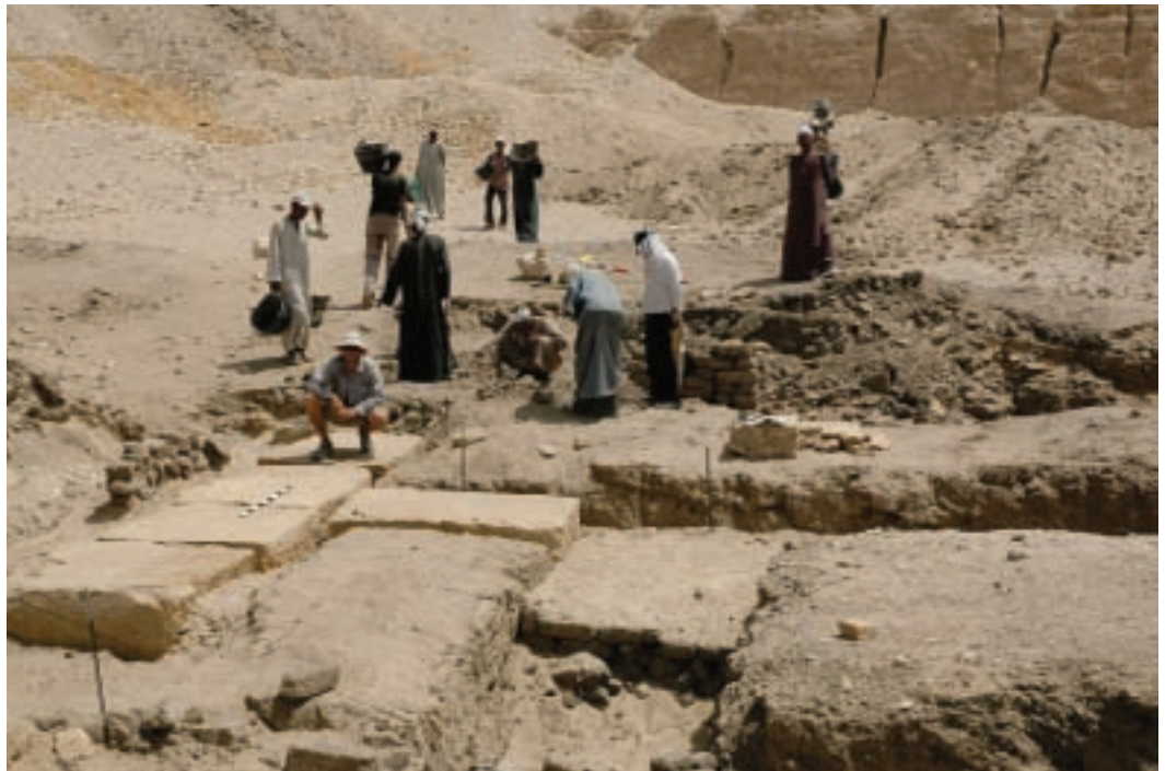
Fig. 7. The first five foundation blocks (still half-buried) beginning to appear in the excavation of trench TB10. Several inscriptions were found on the blocks discovered so far.
