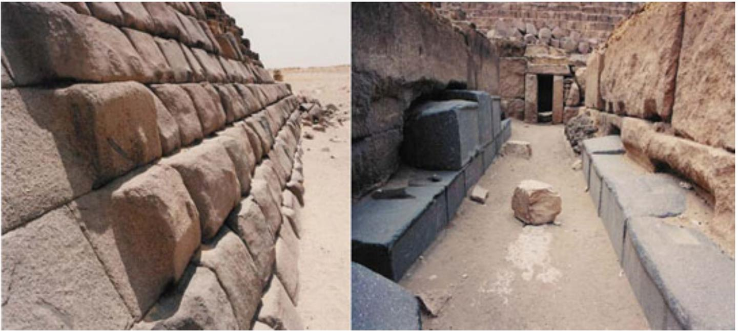
Fig. 2. Left: The granite casing on the northern face of Menkaure's pyramid shows the excess material forming the bulbous face. The material is far more than needed to protect the final, finished face. Right: The dark granite blocks in Menkaure's mortuary temple have prepared faces with only edge protection.
