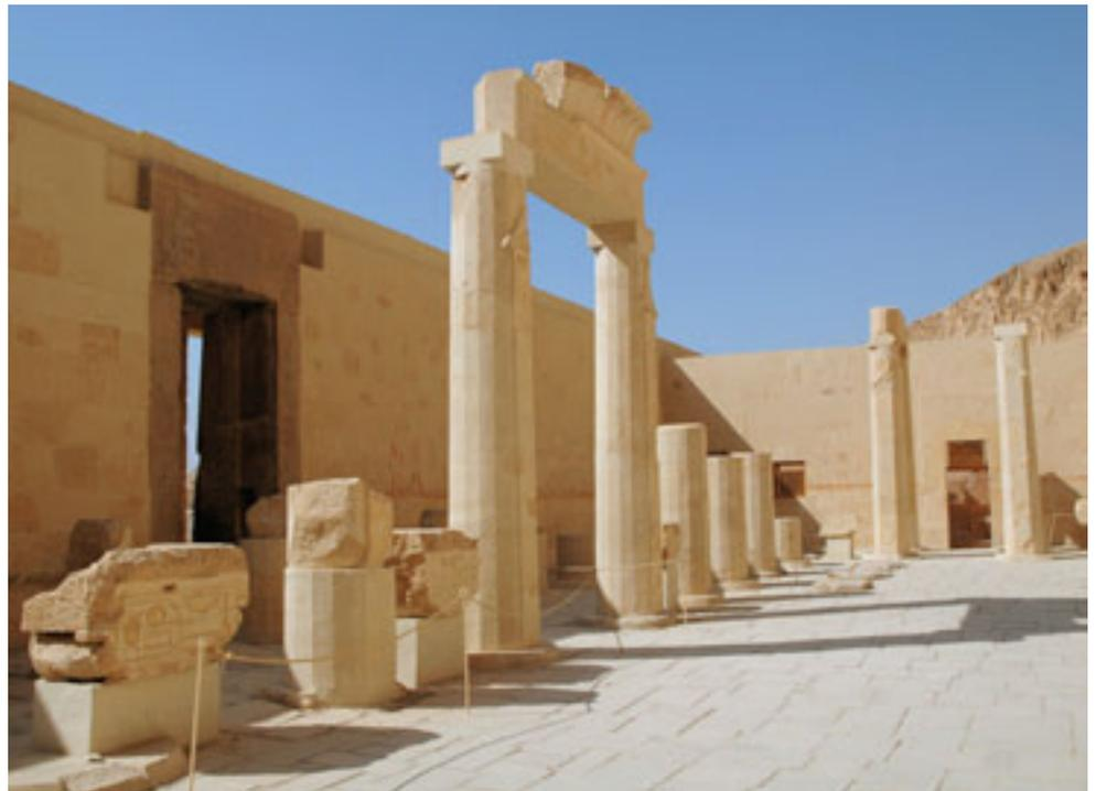
Fig. 1. Upper Courtyard looking towards southeast corner. Polygonal columns have been restored to various heights depending on the number of ancient fragments they contain. Some fragments of architraves are set on plinths (left front).
