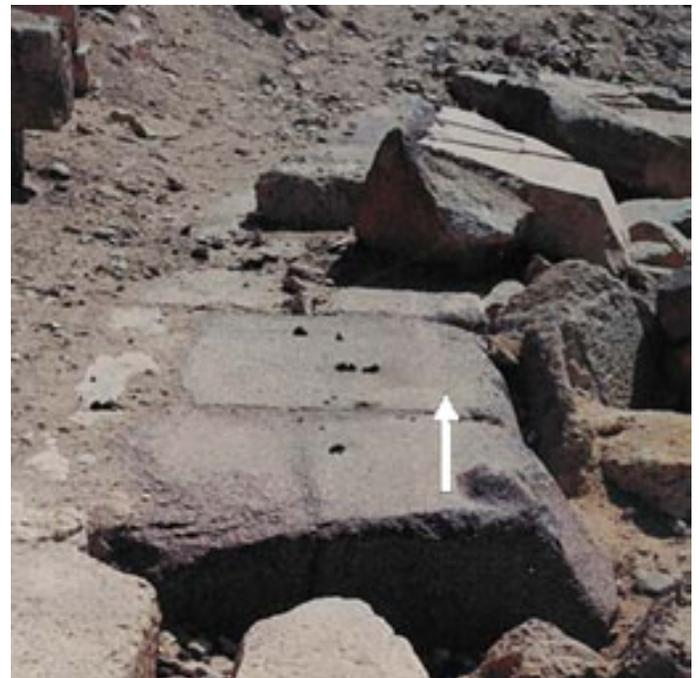
Fig. 3. The granite casing to the south of GIII-a. The pyramid face fell at the arrow; all material to the right was excess.
